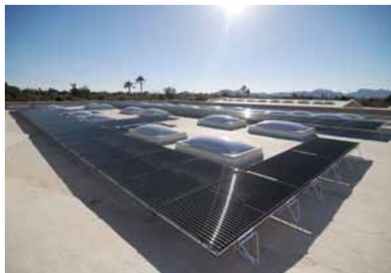
(Top) Dr. Philip Lacovara, with a local television station recording the event, throws the switch to begin using the electricity converted from the sun's rays. (Below) The array of solar photovoltaic panels, located on top of a campus building, which collect the sun's energy. (Photos courtesy of Merri Siler, Salpointe Advancement Office.)
